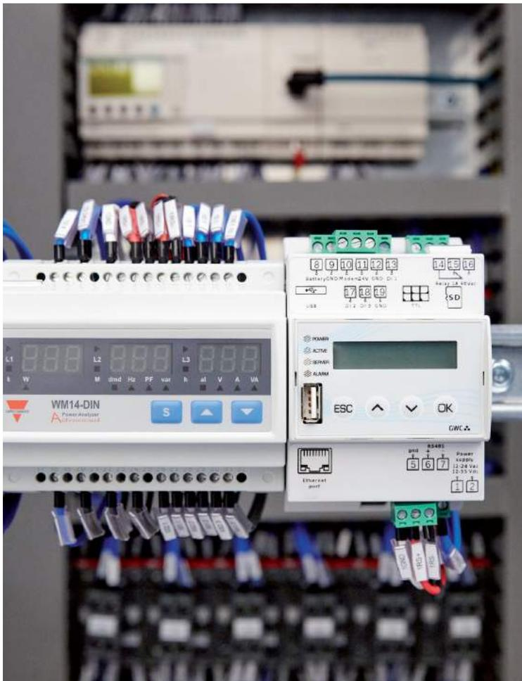
The E-Controller device is mounted inside the control unit of BEGO;
